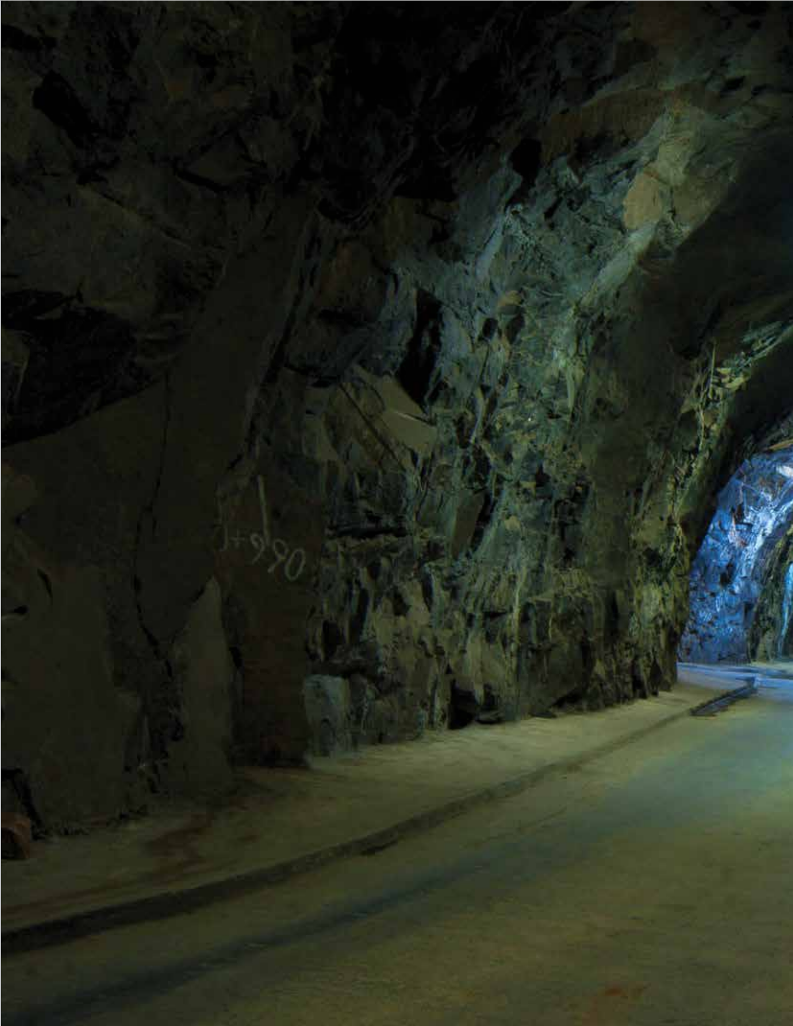
Access tunnel of the 225MW Gitaru Power Station
