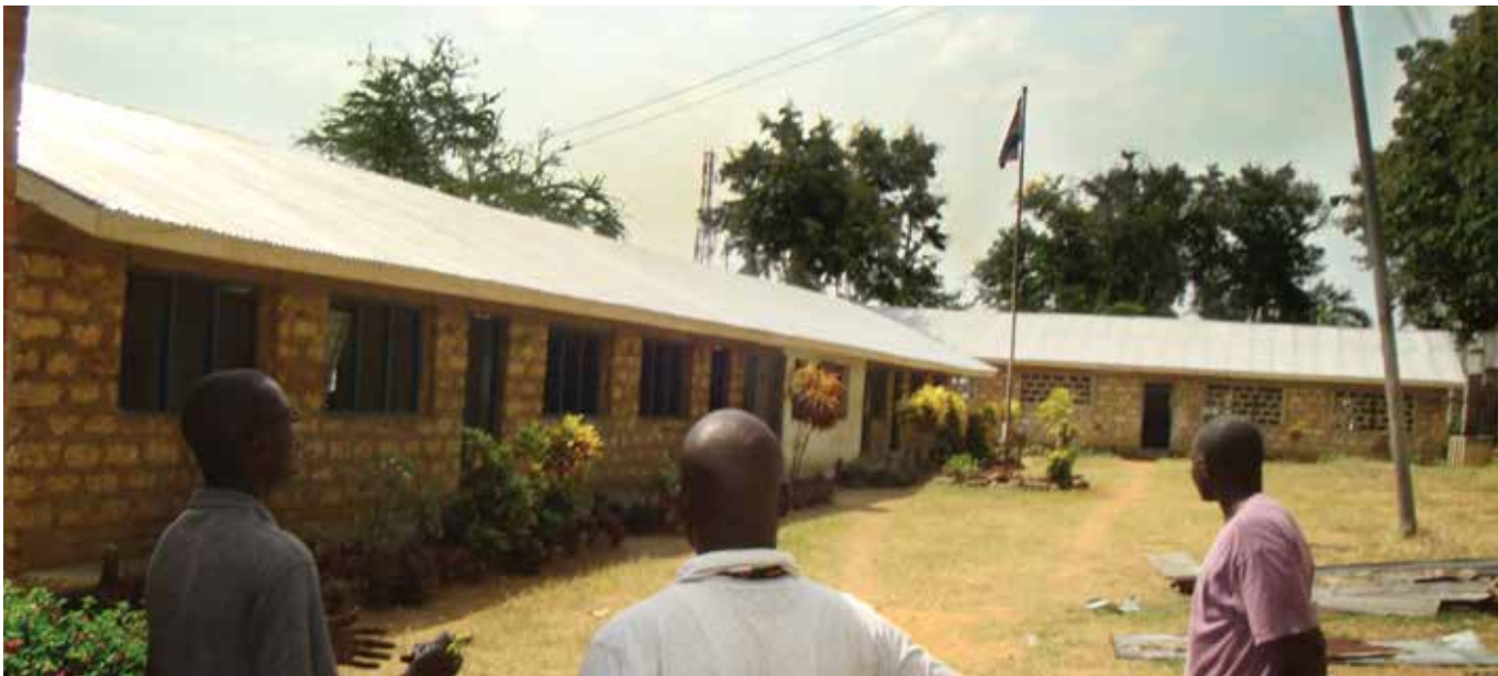
Part of the repaired roof
