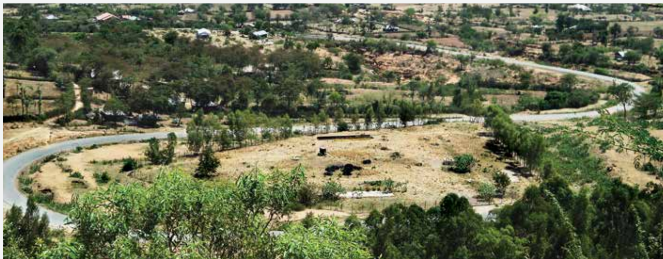
Section of the 6km Sondu - intake road built and maintained by KenGen
