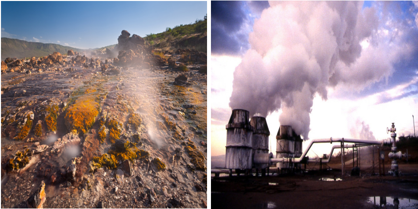
Olkaria Discharging Wells
