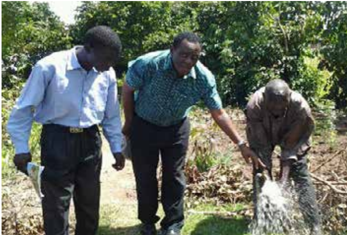
KenGen Foundation Managing Trustee, Mike Njeru test the taps providing running water in Kivaa
