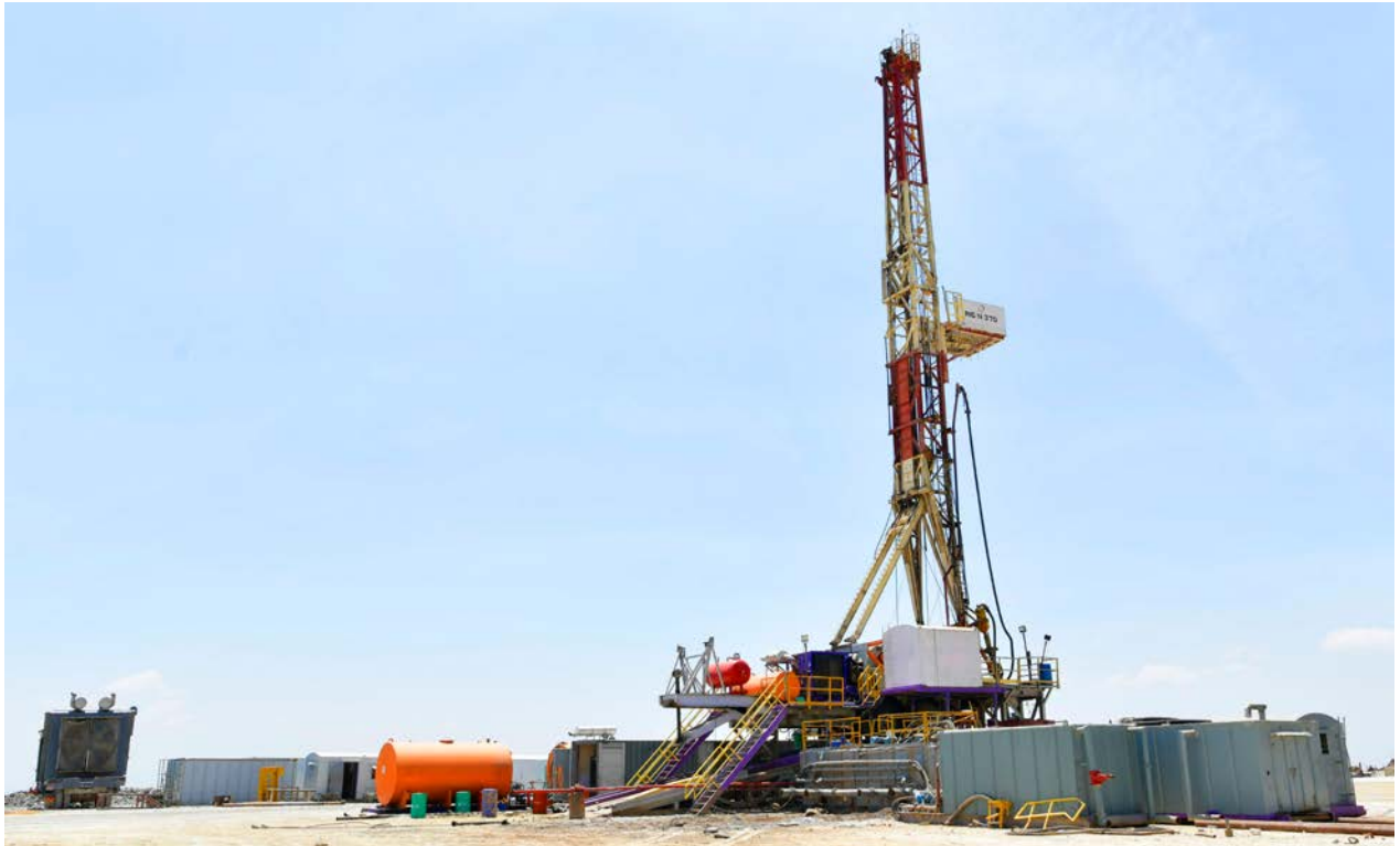
KenGen Geothermal Rig
