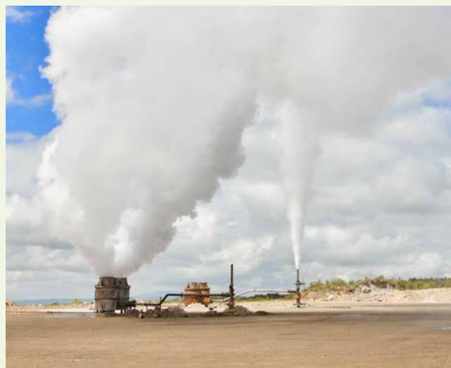
Recently drilled geothermal discharging well
