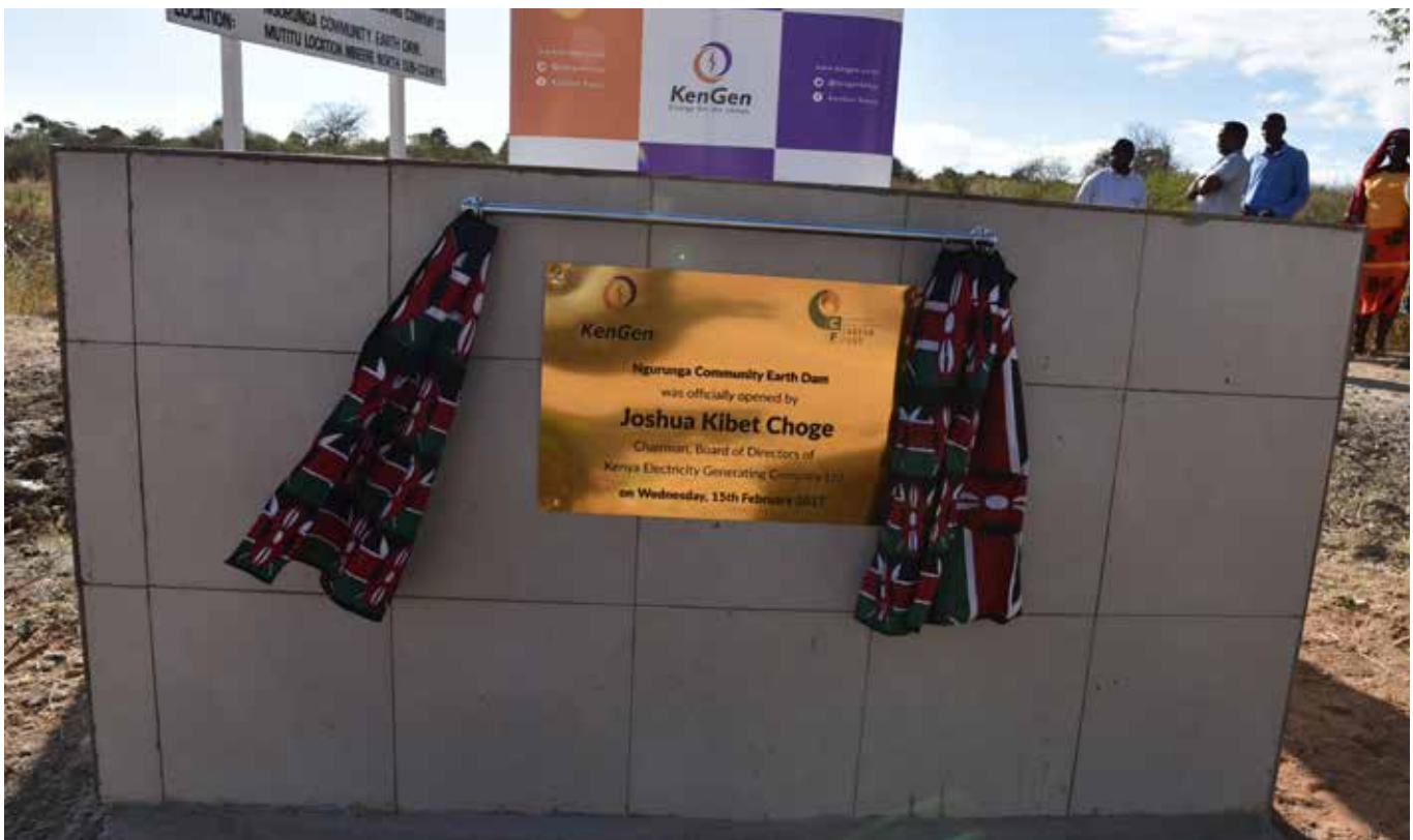
A plaque Commemorating the commissioning of Ngurunga Community Dam
