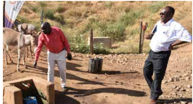
Commissioning of Ngurunga earth water project dam.
