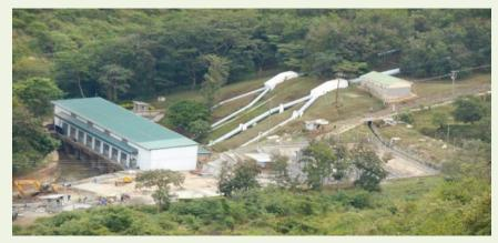
The photo shows the reverbed Wanjii powerhouse, penstocks, winch track and trolly. The evacuation substation was done anew to improve the substation performance. The Winch allows ease of access for staff and equipment to the powerhouse. A road was constructed to the powerhouse to improve access.
