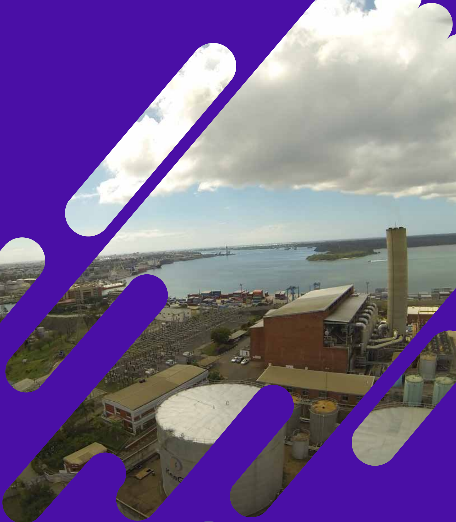
Kipevu Thermal Power Plant, Mombasa
