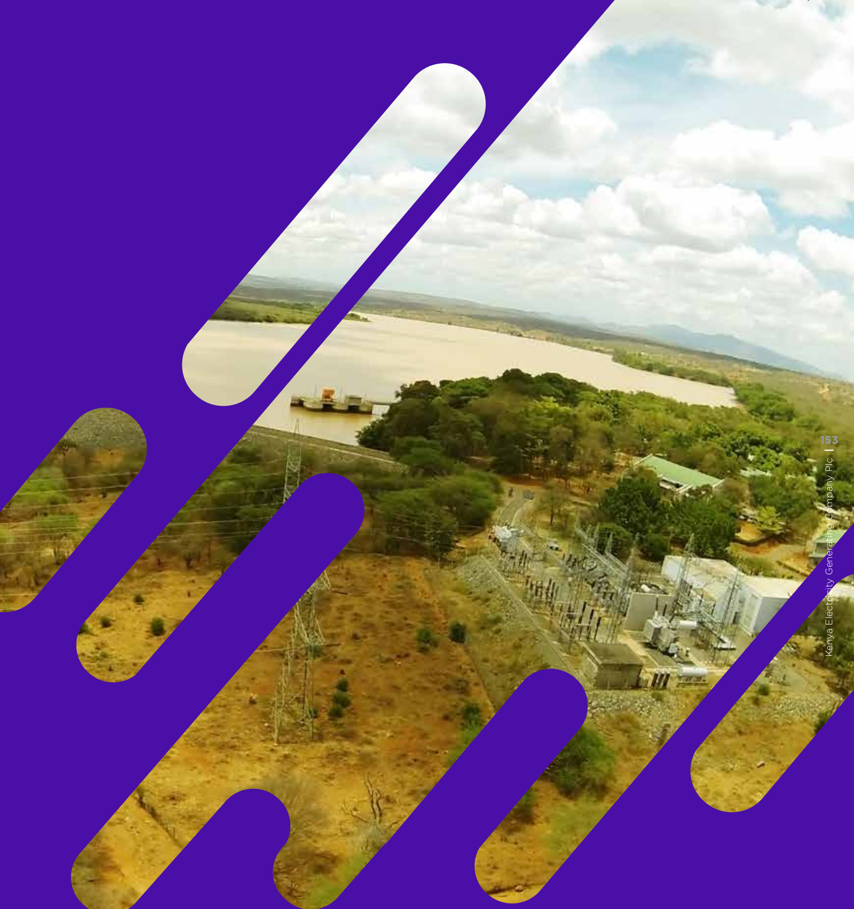
Gitaru Hydro Power Station
