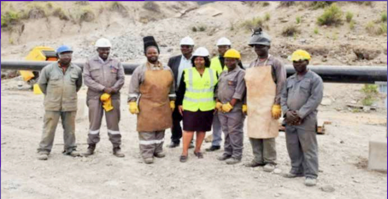
KenGen MD & CEO visits the team that successfully set up steam gathering pipeline at their workplace in the field on March, 2019
