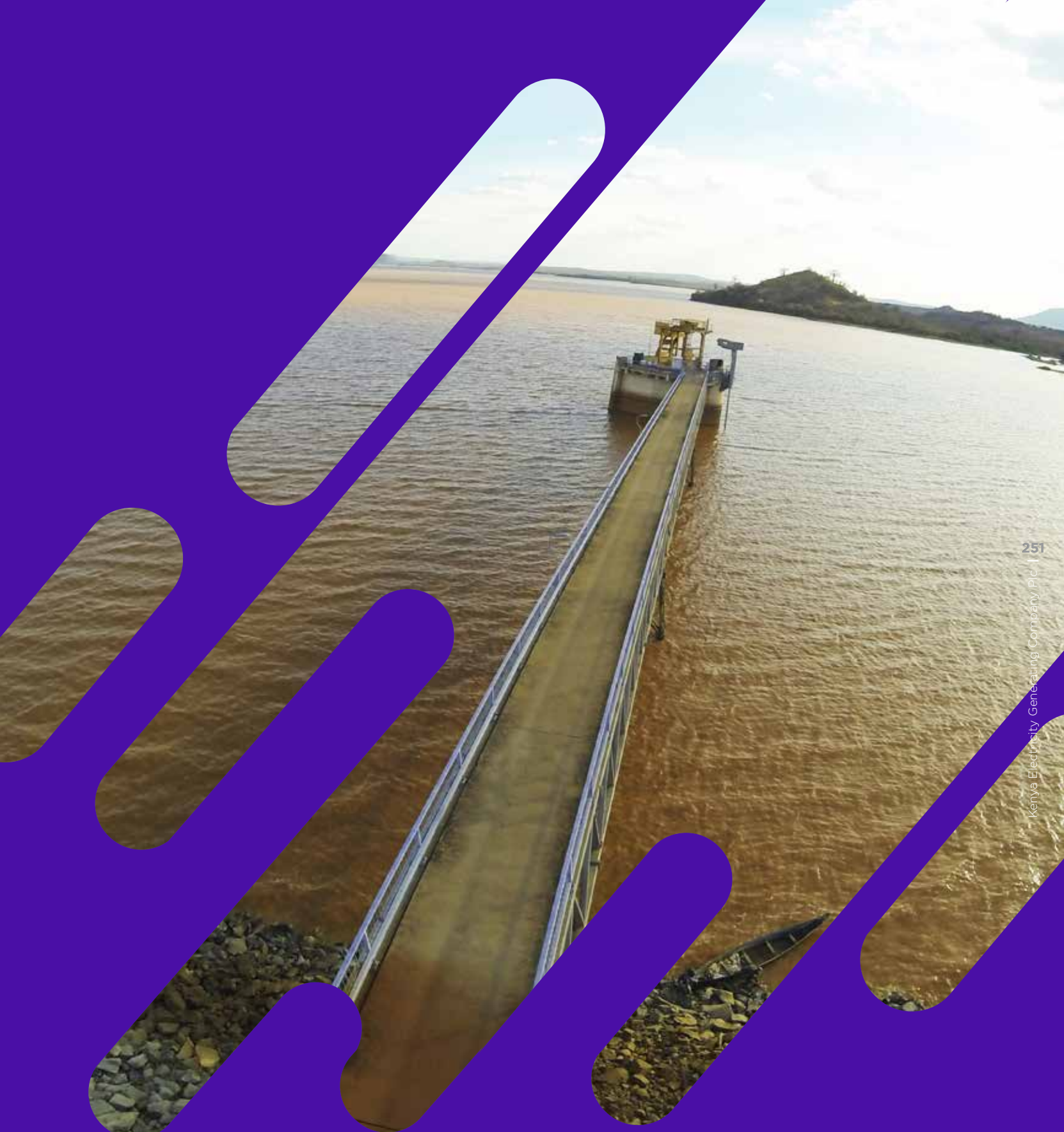
Kiambere Hydro Power Station
