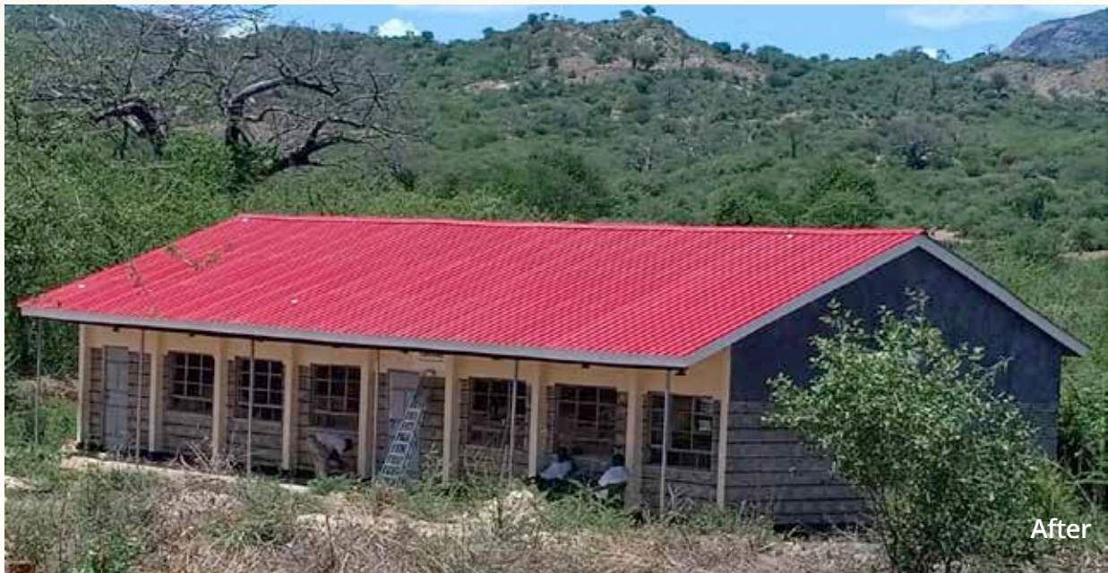
Transformation done by KenGen Foundation at Kiruri Primary School in Mumoni Sub County, Kitui County
