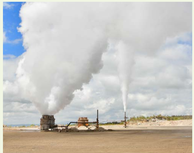
Recently drilled geothermal discharging well
