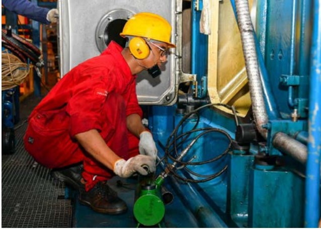
KenGen staff working at Kipevu III Power Station
