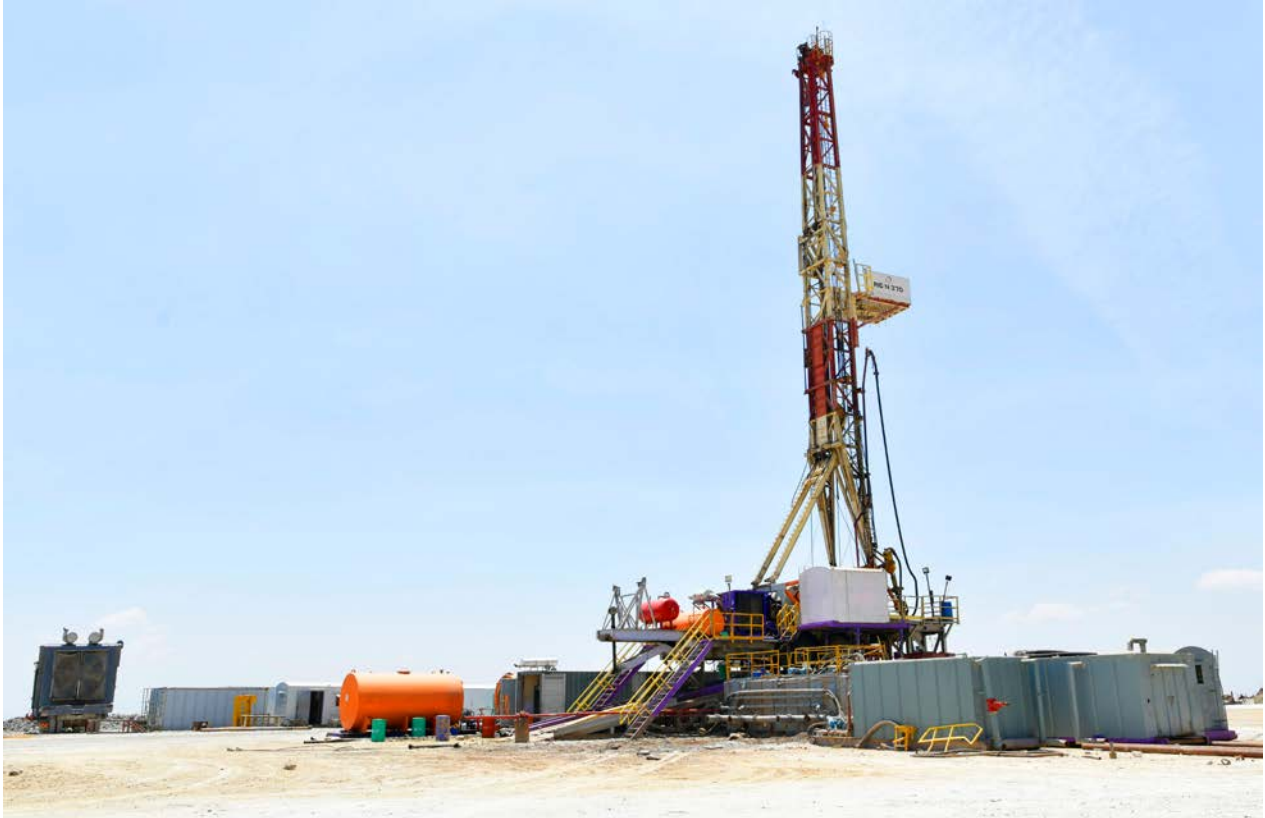
KenGen Geothermal Rig
