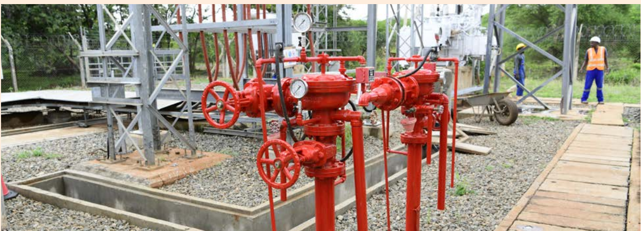
▲ Fire Risk Mitigation at Gitaru Station
