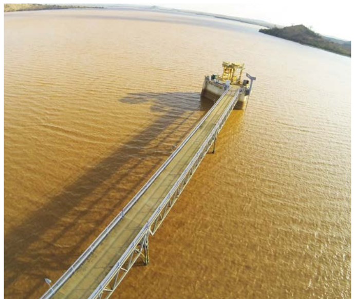
Largest Hydro-powerplant Kiambere 168MW in 2009
