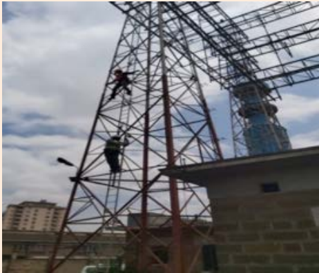
Work at Height Training (WaH) ▲
