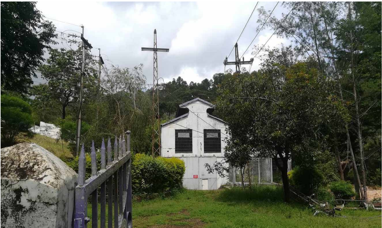
Decommissioned Ndula Hydro Power Plant now Ndula Museum
