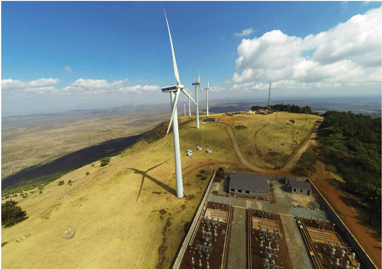
Ngong Wind Farm
