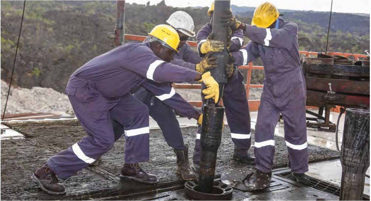
KenGen Team working on Olkaria V project
