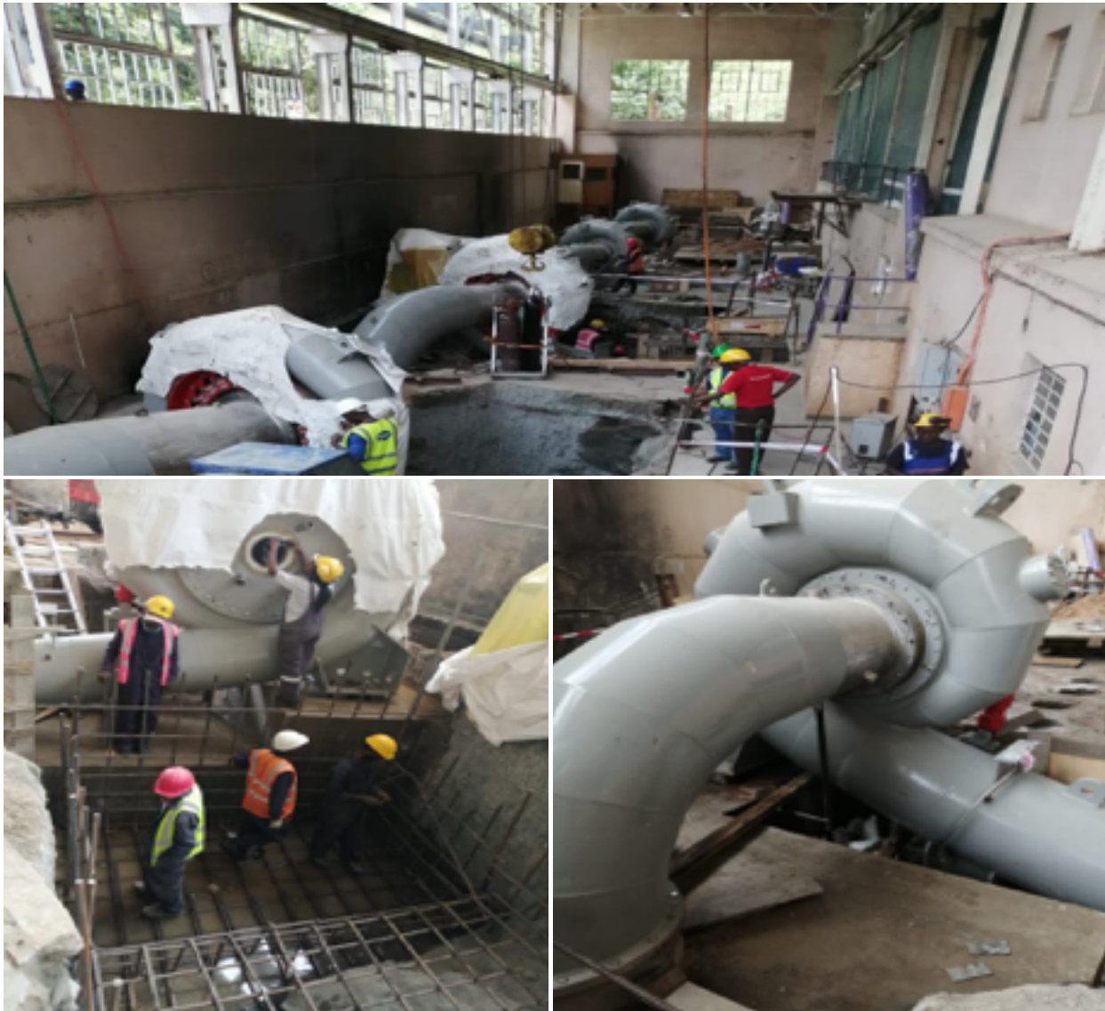
Rehabilitation works at Wanjii hydro power station by KenGen staff and Voith consultant
