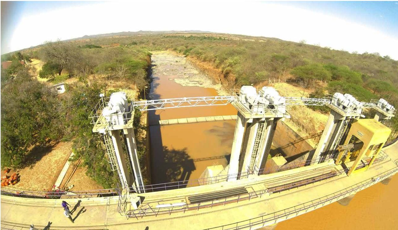
Kindaruma reservoir spillway
